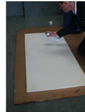
Spray adhesive all over the drum.
